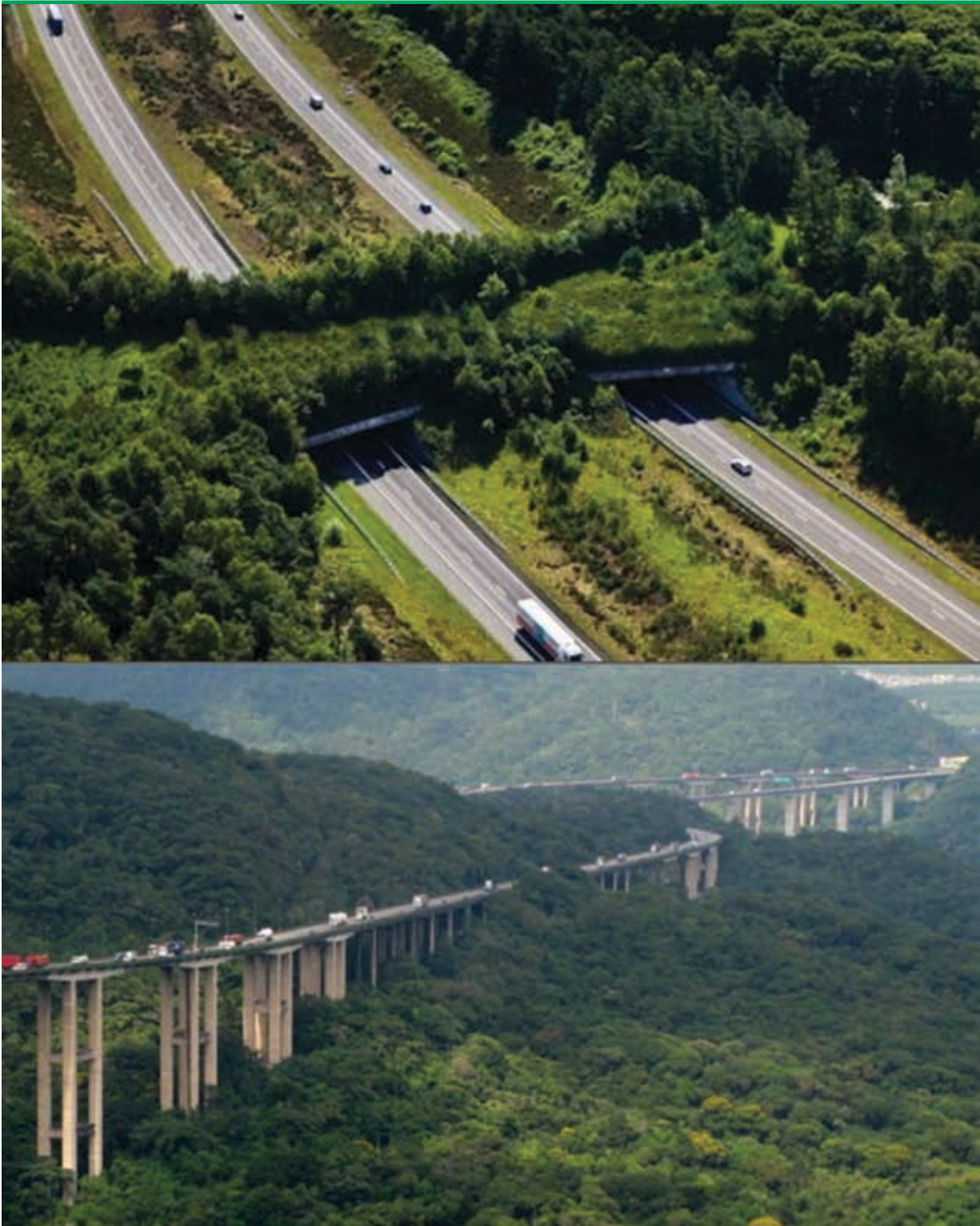
Figure 10. Overpasses and underpasses that allow integration of roads with wildlife crossings. These kinds of infrastructure can be used in planning for Grey and Green infrastructure. Photocredits: top: Ecoduct – Wildlife Bridge – the Netherlands alizul2 blog. Bottom: http://io9.gizmodo.com/5989331/how-well-live-in-a-future-where-cities-have-become-forests
