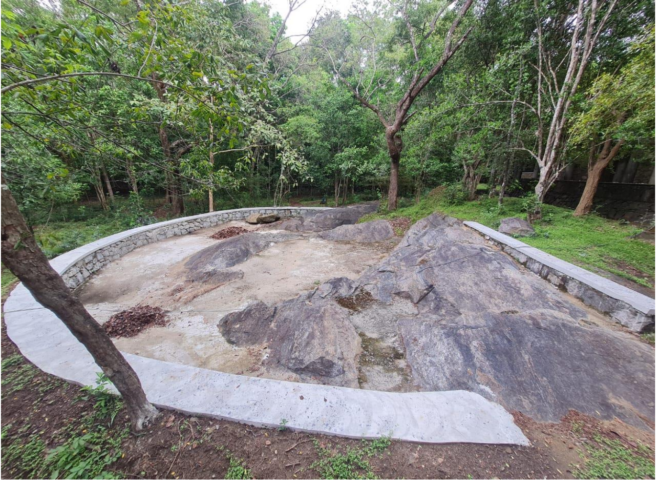
Improved the facilities for the open lecture area
