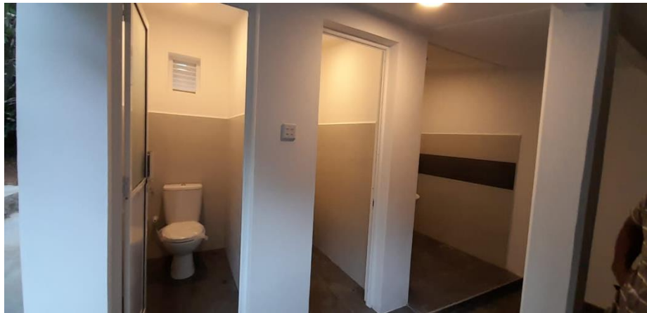
Constructed new toilets
