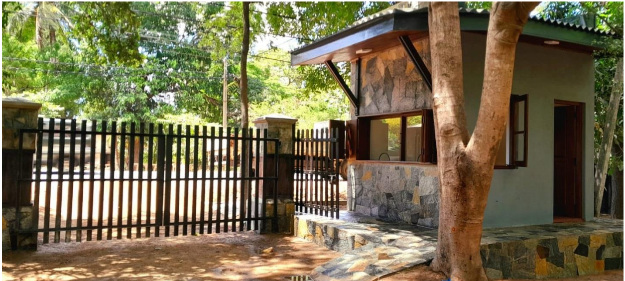
Constructed the ticket counter
