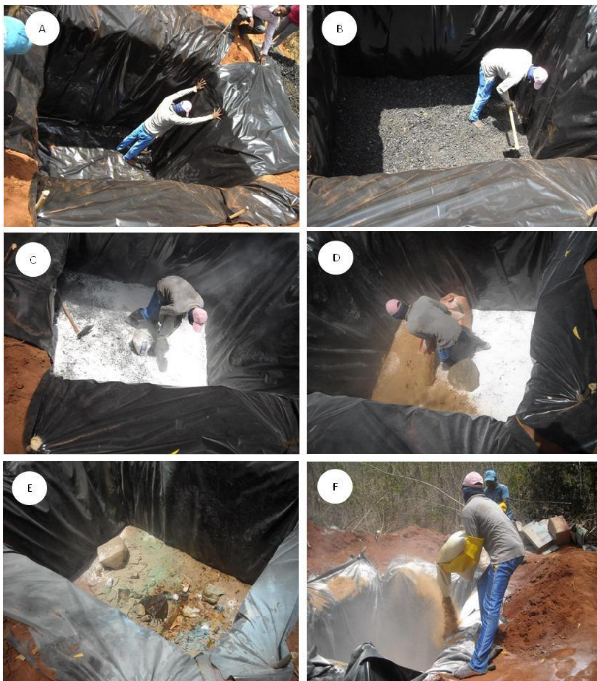
Figure 4: The practice of ground burial of obsolete non-POPs pesticides at farm level approved by the Pesticide Authority, Sri Lanka; Date of treatment 20.10.2014 at Wanathawilluwa. (A) Lining of the burial pit with polyethylene; (B) Filling charcoal layer; (C) Filling lime powder layer; (D) Filling saw dust layer; (E) Obsolete pesticides and waste materials; (F) Filling covering materials. (Photos by W. Gunawardena).
